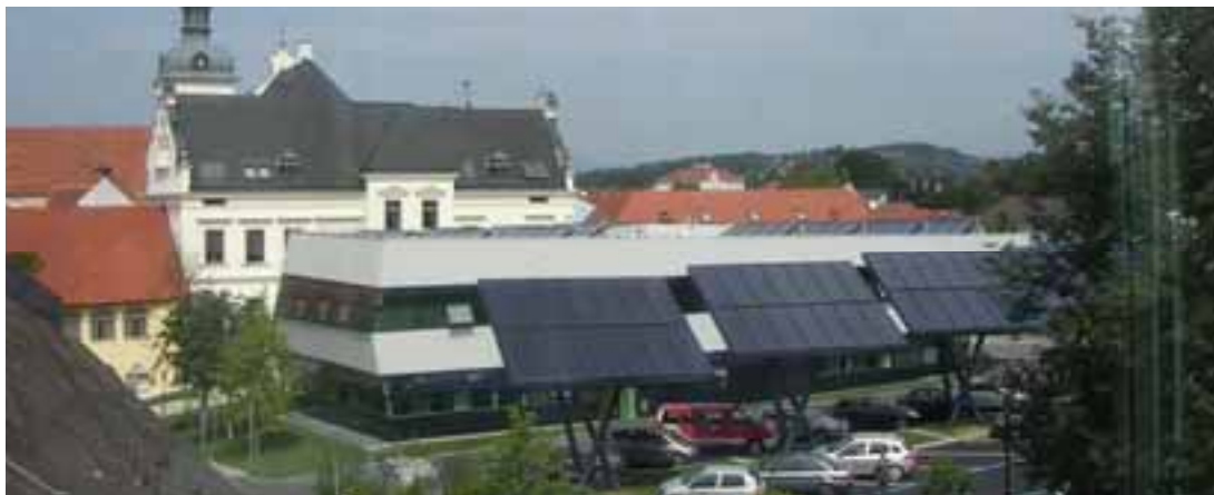
Figure 1: Photo of the old renovated Town Hall and the newly built Service Centre (source: AEE INTEC)
