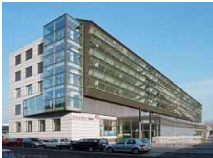
Figure 4: Photo of newly built ENERGYbase building (source: Wiener Wirtschaftsförderungsfond)
