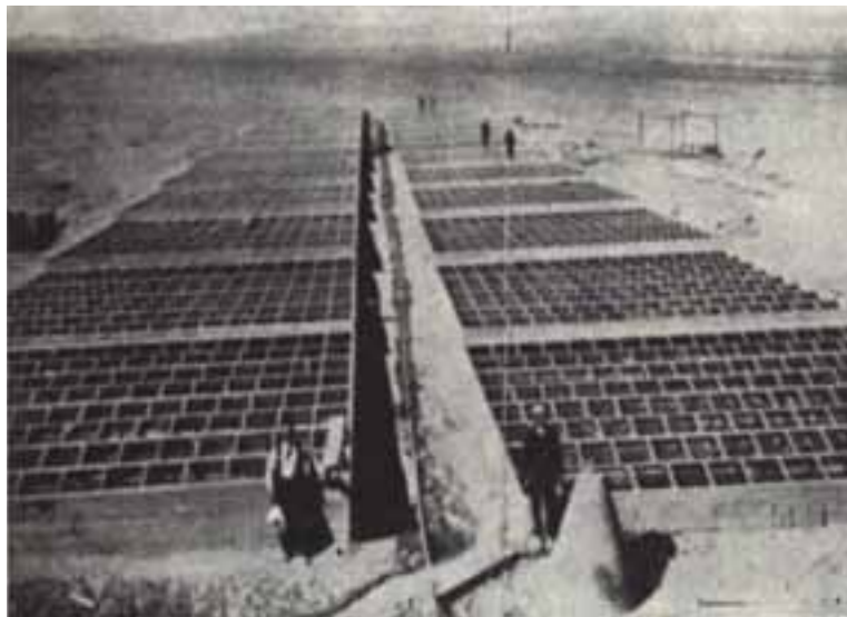
Fig. 1 The Las Salinas Solar Desalination Plant. Photograph from [1], taken around 1912
