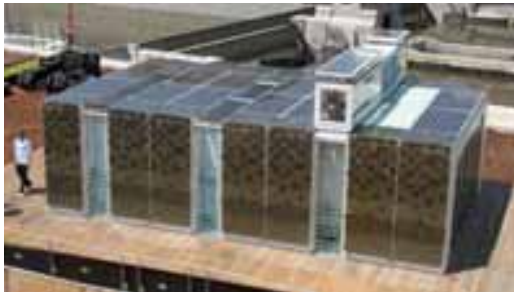
Fig. 6: The solar activated power envelope of Stuttgart's home + in Madrid (Source: Jan Cremers)
