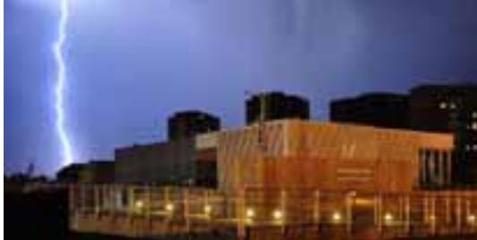
Fig. 4: View to the north-east façade with the terrace (Source: Oliver Pausch)
