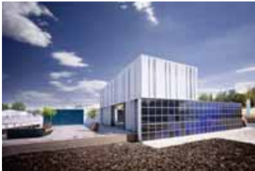
Fig. 8: View to the south facade with PV wall (front) and vacuum tube collectors (back).
