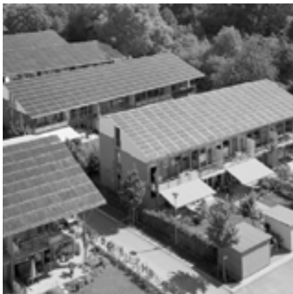
Fig. 1. Monitored Net Plus Energy Settlement, Freiburg, Germany [2]
