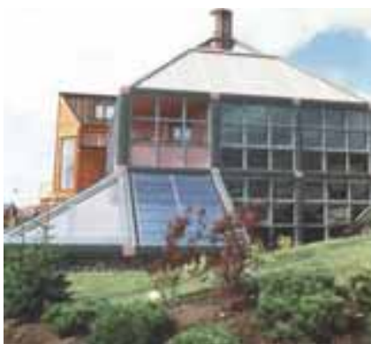
Fig 1. Chanelle. Europe's first modern time's ZEB? Designed 1985. Completed 1988 (RøstvikAS)
