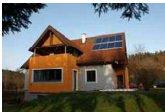
Fig 2. Example of a detached house in Austria with 16 m 2 collector area
