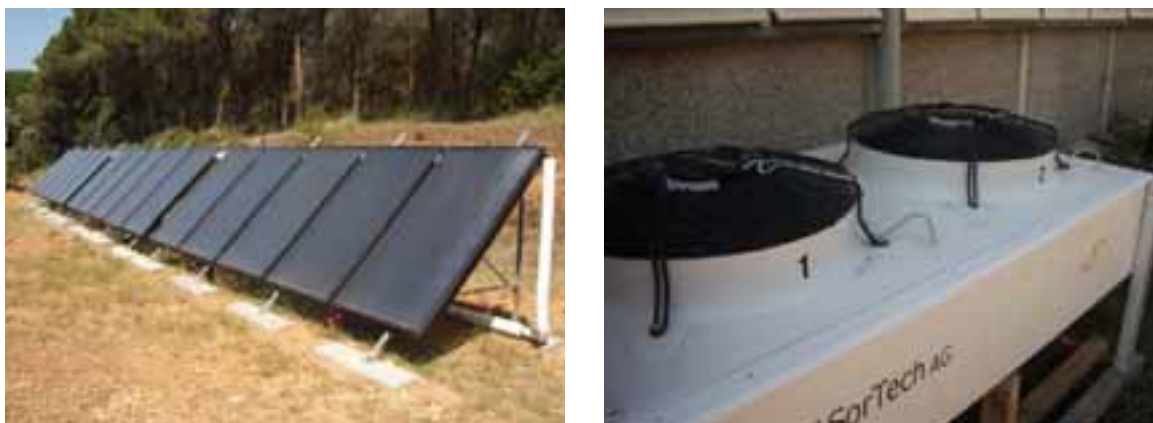
Fig. 1. Air conditioning solar plant. Left: Collector field composed by 15 Maxol 2.0 S units. Right: RCS 08 SorTech re-cooling system.
