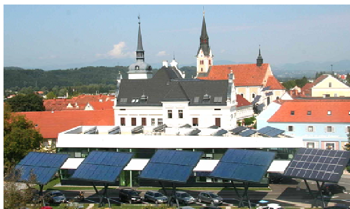
Fig. 2. In the foreground 4 Solar Trees and 1 PV tree, behind the Service Center with roof collectors and in the background the Town Hall (source: SOLID)
