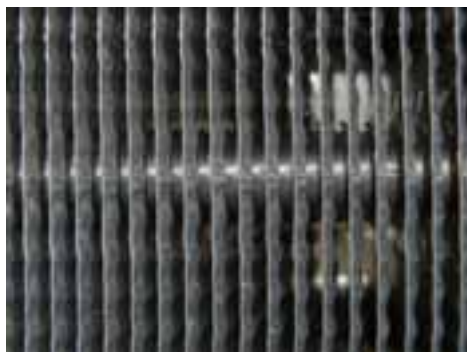
Fig. 4: Sector of the lamellas of the dry cooler heat exchanger. In the middle one of the fluid carrying pipes can be seen. The corrugated aluminum lamellas have a thickness of 0.2mm.
