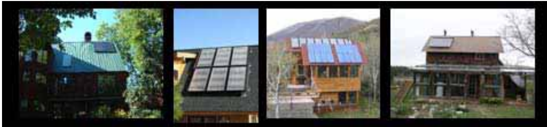
Fig. 1 Solar collectors randomly mounted on roofs.
