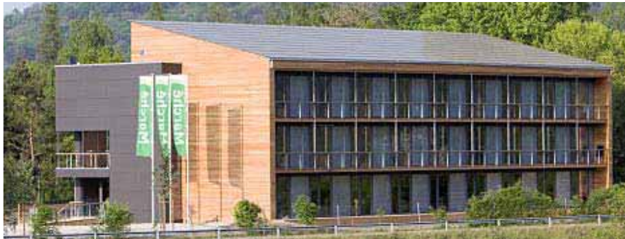
Figure 5: PV installation generally acknowledged as well integrated. Marché International Support Office in Kempththal by Beat Arch. Kämpfen. Source: Kämpfen für Architektur
