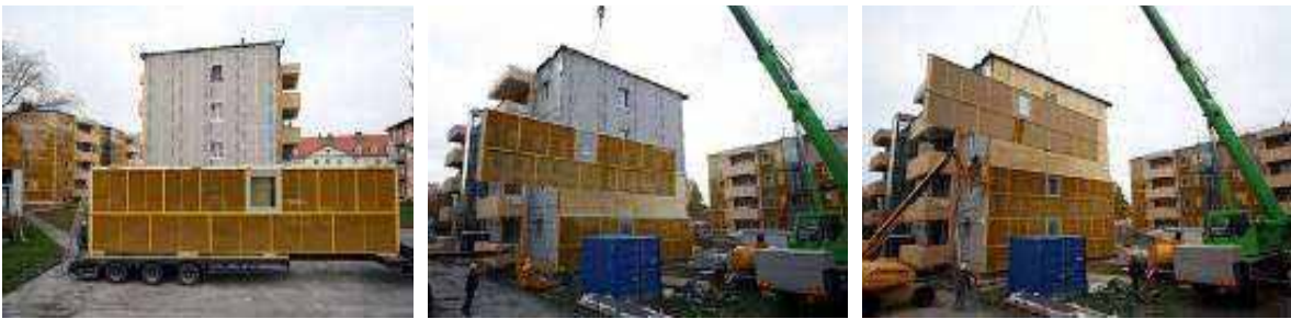
Figure 4: Transport on-site and assembling procedure (Source: gap-solution)
