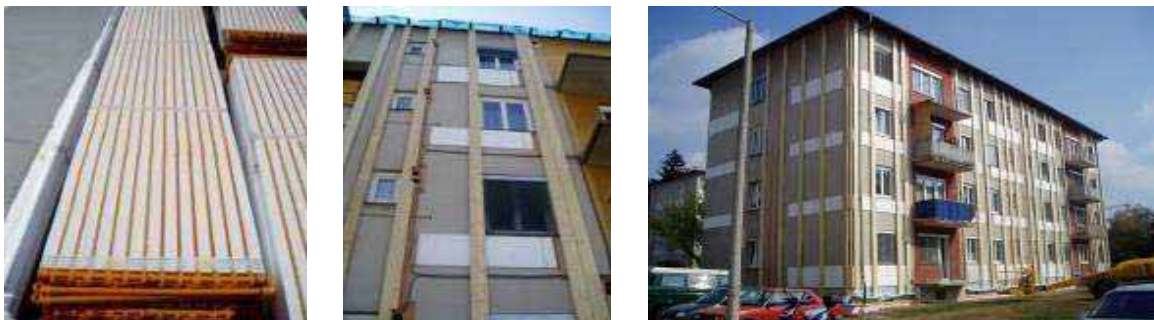
Figure 7: Heat dissipation system installed on the outside of the exterior wall (Source: AEE INTEC)
