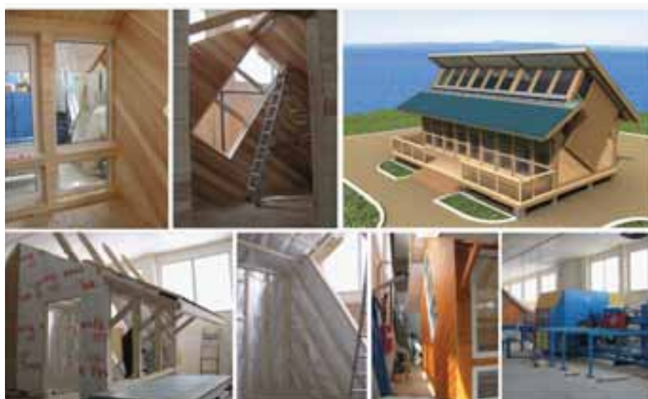
Fig.5. “EcoModule Solar-5M” under construction in “Technopark” FENTU.
