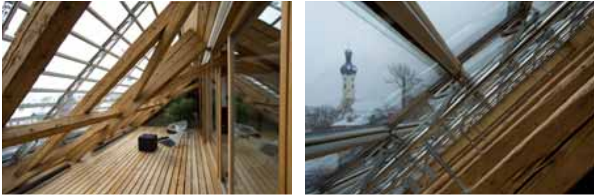
The loggia in the solar roof
