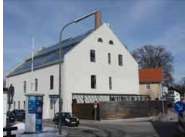
In 2008 after renovation
