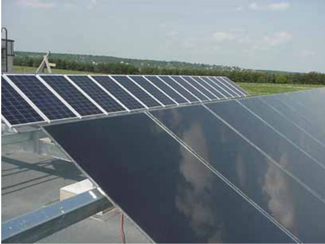
Fig.1. Polycrystalline (back) and amorphous silicon (in front) PV modules.
