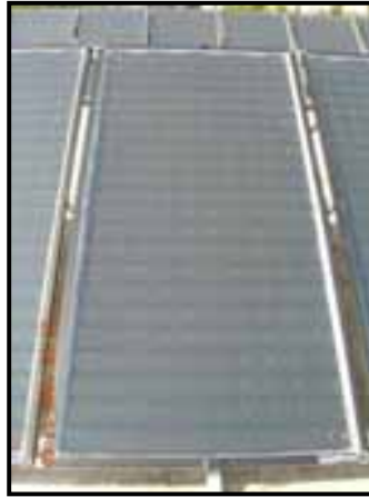
Fig. 2. Solar vacuum flat plate collectors in the Solar Experimental Plant (CSIC).
