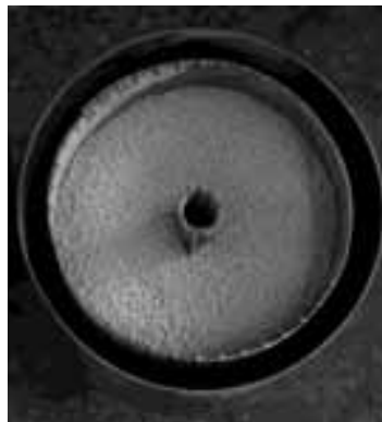
Fig. 5. View from top into radial flow adsorber filled with zeolite (top cover removed)
