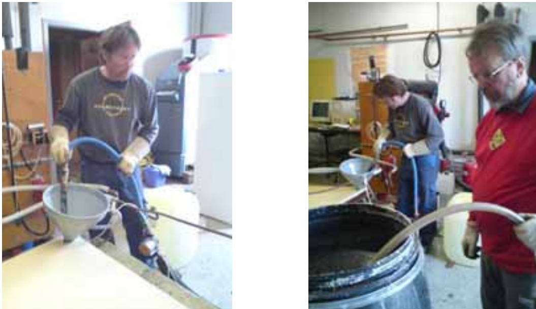
Fig. 5. Salt water mixture from a plastic tank pumped into a heat storage module.
