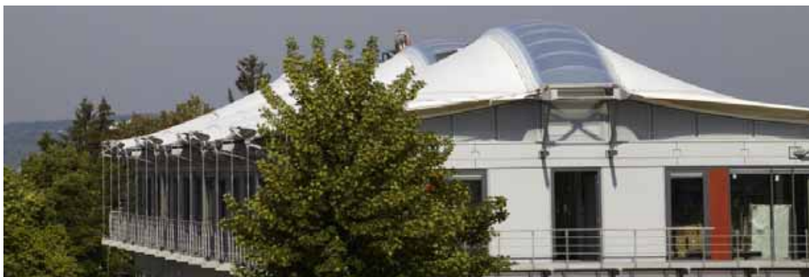
Fig. 1: Energy Efficiency Center viewed from south-east. Clearly visible is the textile roof with translucent PTFE-glass membranes and partially transparent ETFE films.
