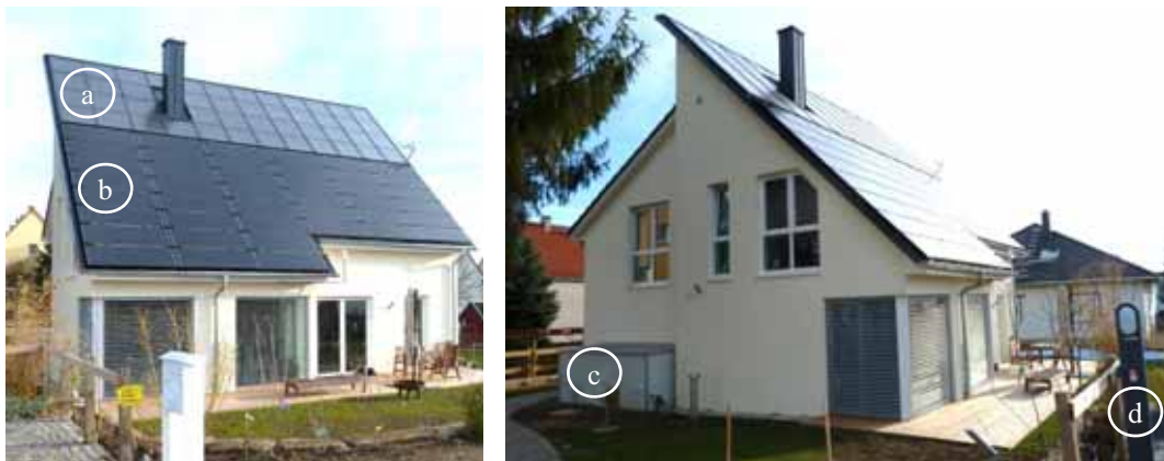
Fig.2: Occupied energy-autonomous house with roof integrated solar collectors (a), pv panels (b), storage battery (c) and charging column for electro mobility (d)
