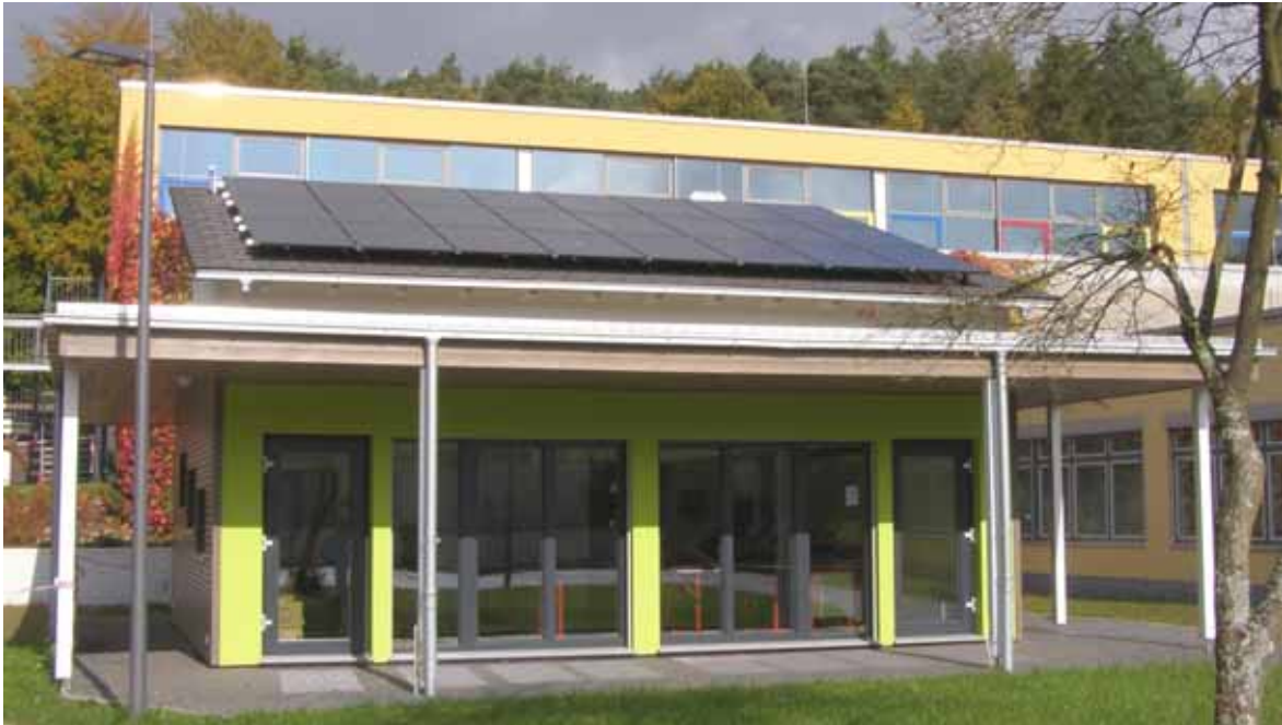
Fig. 1: front view of the school building
