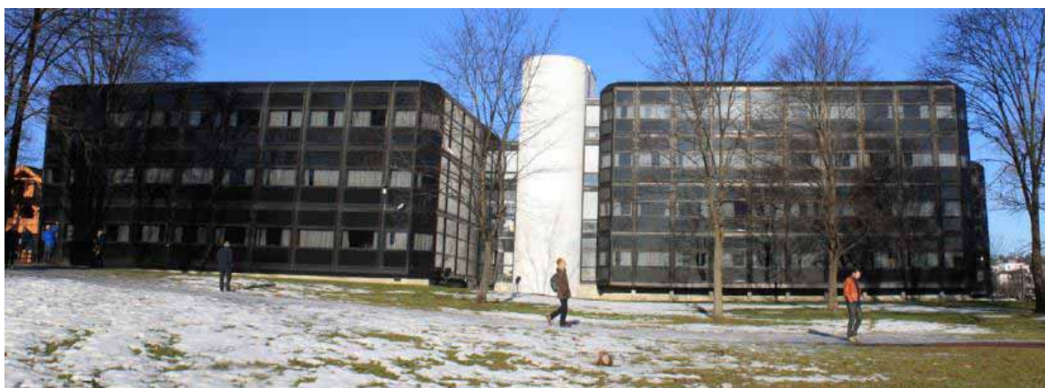
Figure 1: Office buildings before refurbishment
