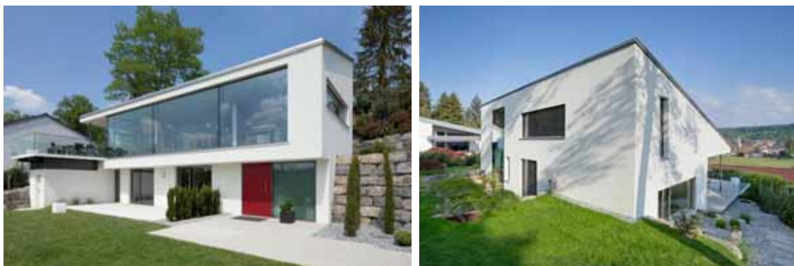
Fig. 1: South side with cantilever as structural sun protection (left), north-west side (right)
