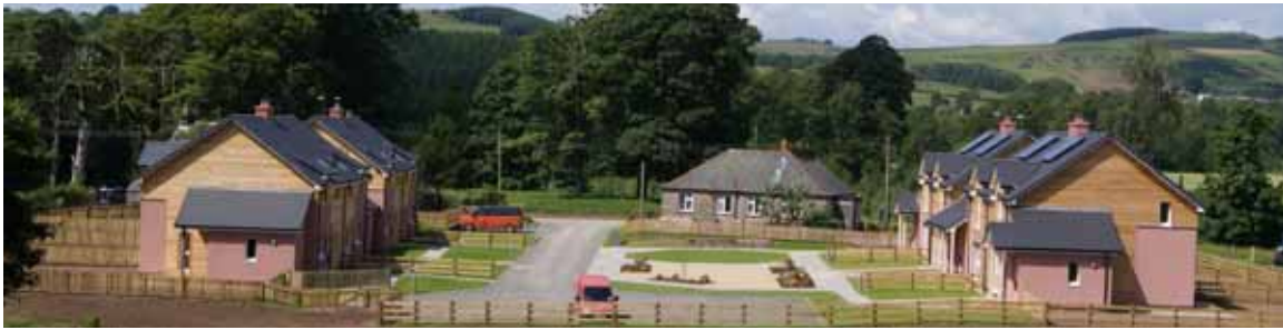
Fig. 1: Overview of the 8-house development from the East, showing the shared courtyard and rural setting.
