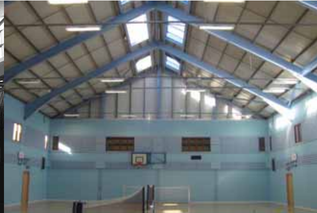
Figure 6b: Internal view of the main hall at Sporsnis. Borrowed daylight from the first floor gallery enters the hall through high level glazing (left of image). While the roof lights allow natural daylight. (The daylight sensing for the artificial lighting system was still to be commissioned at the time of the photograph).
