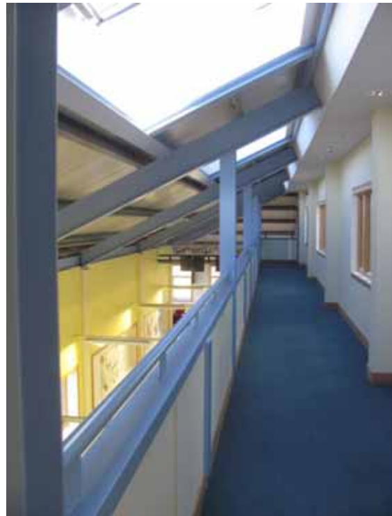
Figure 5: Internal view of first floor gallery, roof lights provide daylighting to gallery and ground floor. The windows on the right allow borrowed daylight in to the main hall.
