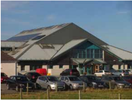
Figure 1a: External view of new-build community resource, Sporsnis, Ness, Isle of Lewis. Solar PV array, solar thermal and rooflights visible from higher ground near the site.
