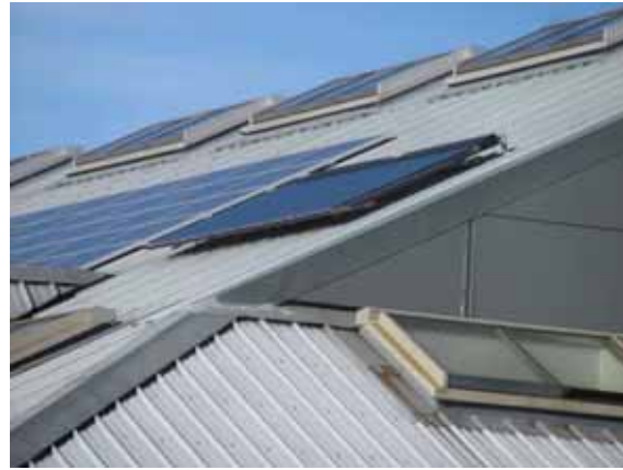
Figure 1b: Roof of new-build community resource, Sporsnis, Ness, Isle of Lewis, indicating building added PV, solar thermal and rooflights.
