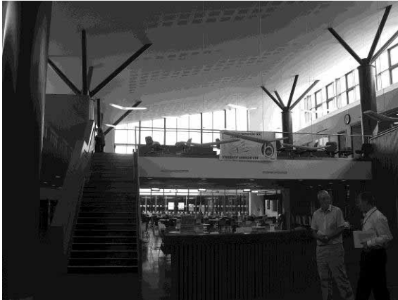
Figure 6a: Internal view of Banff and Buchan College, daylit using high level clerestory (right of image) and glazed façade.
