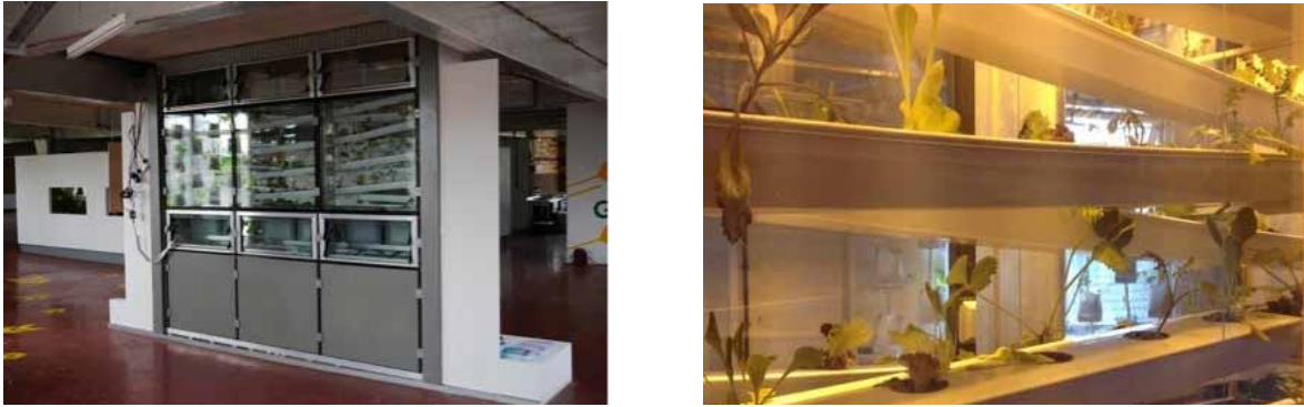
Fig 8: Single bay prototype of facade farm with view showing internal crop growth
