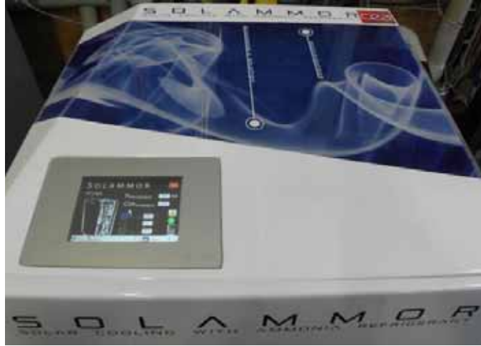
Fig. 4: Touch screen to control the chiller
