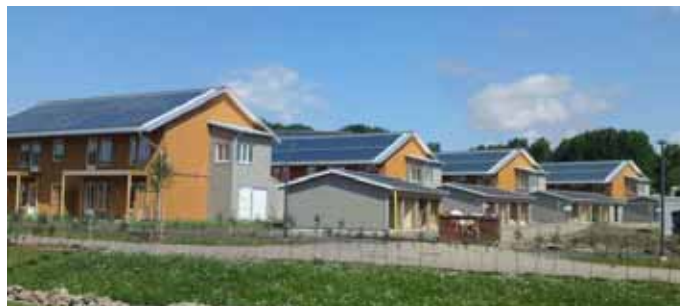
Fig. 2: Multifamily buildings with roof-integrated solar collectors
