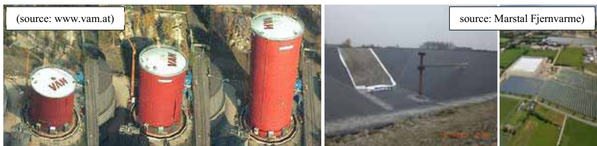
Fig. 1: (left) Buffer TES of the district heating system in Linz. (middle/right) pit heat store in Marstal (sunstore IV)
