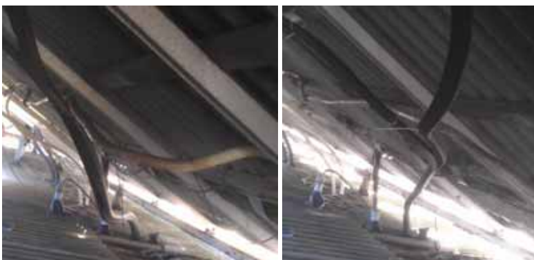
Figure 1c. The collector loop stainless steel flex pipes in the lab system , before and after slope adjustment.
