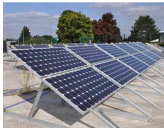
Figure 3 : Experimental set-up to evaluate the concept of PV DHWS
