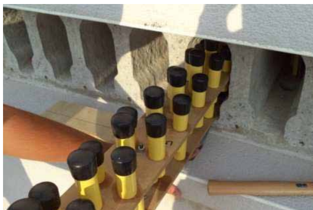
Fig. 2: Incorporation of PCM macro-encapsulated in aluminium tubs inside concrete slab
