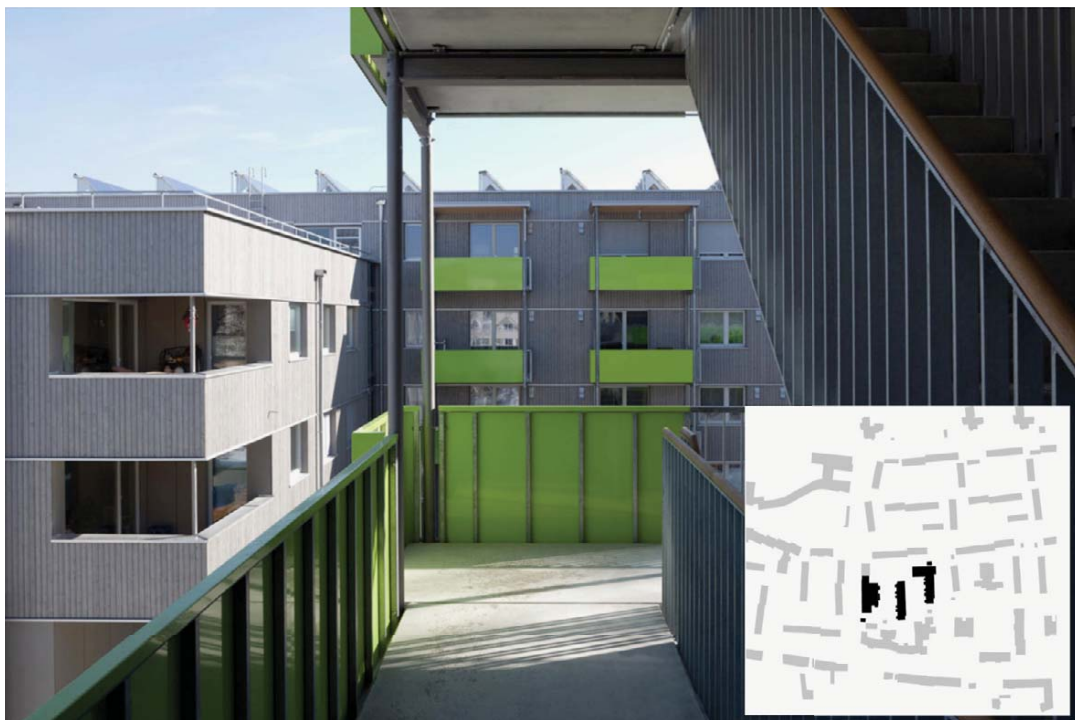
Fig. 1: Renewal post-war housing estate Munich, arcade view to the East, phase 1
