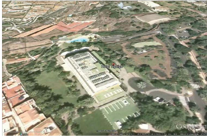
Fig. 2: Top view of the hotel with the solar thermal collectors on the roof (GoogleEarth).
