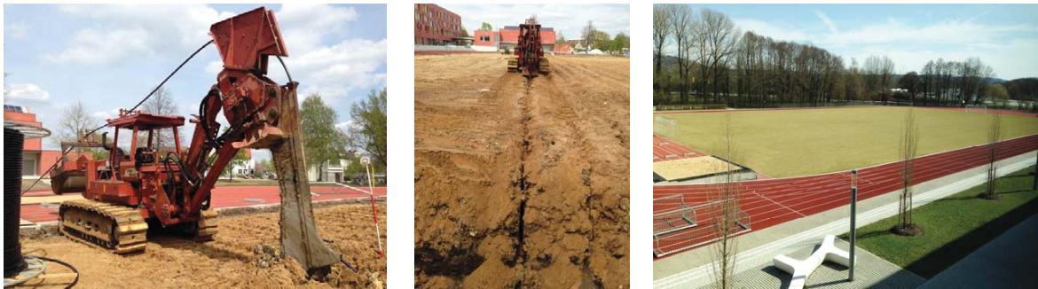
Fig. 7: Ploughing with pipe installation and completed sports field including the pipes
