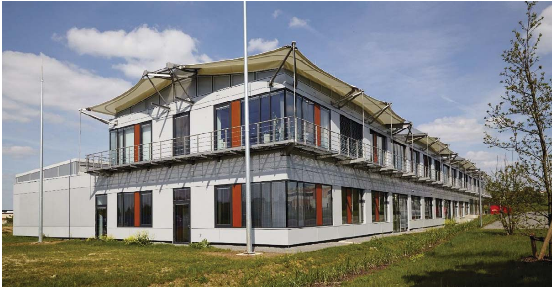
Fig. 1: South-west view of the Energy Efficiency Center in Würzburg. © ZAE Bayern, photo by Petra Höglmeier.
