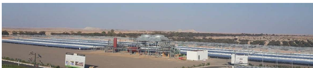
Fig. 1: Picture of the 1MW CSP-ORC plant under commissioning in Benguerir, Morocco
