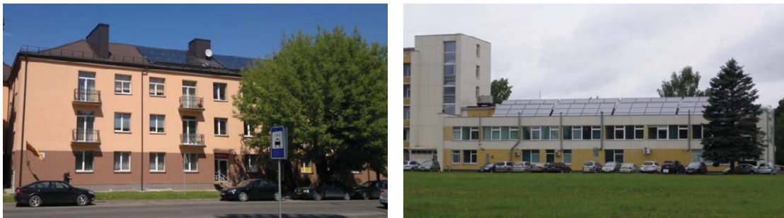
Fig. 1: The first solar thermal system 60 m 2 in multi-family building in Panevėžys city and the biggest solar thermal system 204 m 2 in Plungė town hospital (till the end of 2015).
