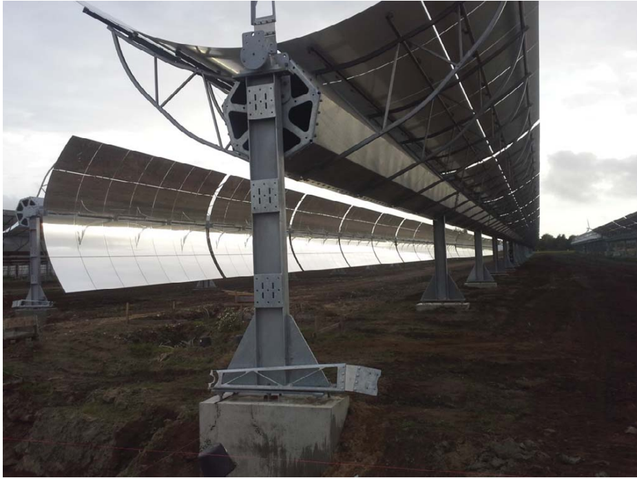
Fig 3. Photo of the CSP collector field, under construction. The collector rows are 240 m long and a total length of 480m of collectors are series connected in each series loop. (No absorbers or connecting pipes are installed in this photo).
