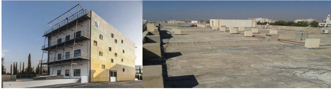
Figure 1. Novel Technologies Laboratory (left), rooftop of the University College in Irbid (right)
