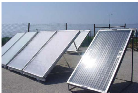
Fig. 1: Installation of collector in OET- Maritime/Industrial
