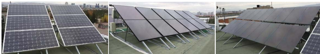
Fig. 1: Mono-Si, micro-crystalline based amorphous silicon and CdTe grid connected PV systems.
