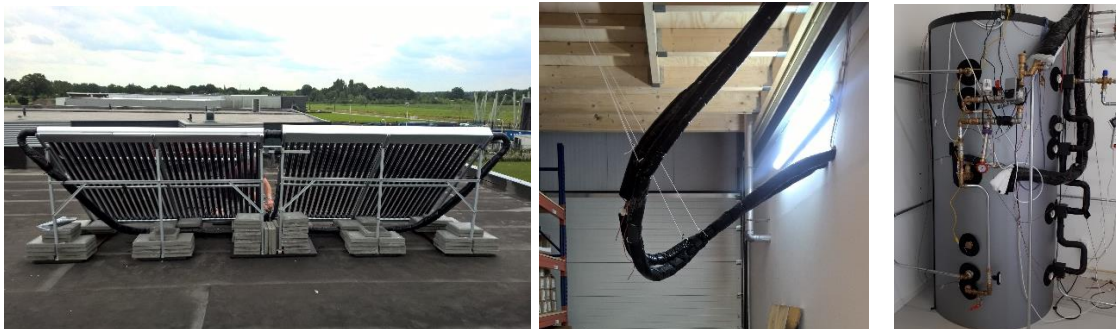
Fig. 6: Images of direct solar system with TDBV; collector array (left), adjustable negative loop (middle) and the storage tank (right) with TDV installed at 0.5 relative height, and thermostat valve at 0.8 relative height
