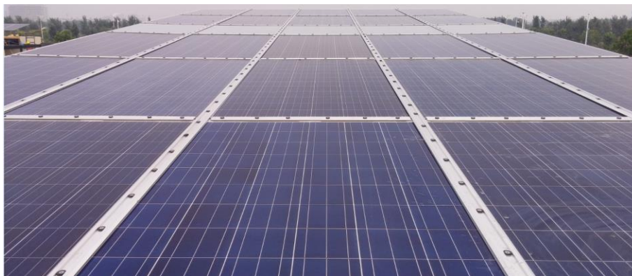
Fig. 5: Finished BIPV/T roof with integrated skylight
