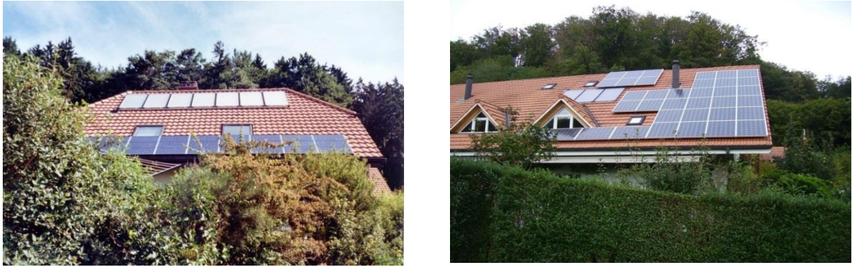
Fig. 6: Typical houses of a solar energy consumer around the year 2005. The hot water solar thermal device (left picture) cost about 15'000 sFr. (or US$). The 6 kWp PV plant (right picture) was about 50-60'000sFr. (Photos: Muntwyler).
