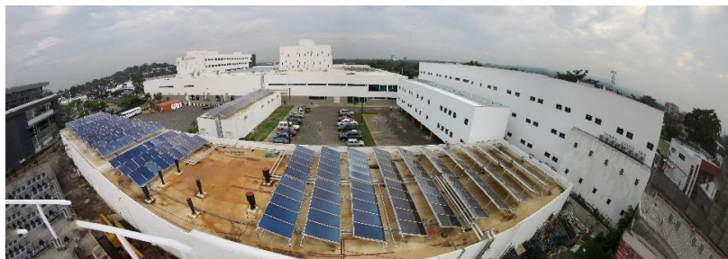
Fig. 4: Panorama view of 4450 m 2 collector area installed at Managua Hospital, Nicaragua.
