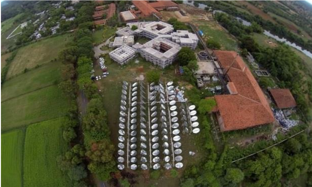
Figure 5 Aerial view of the cancer hospital with solar assisted cooling system
