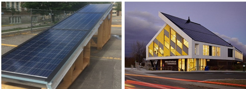
Fig. 2: Modular BIPV/T prototype for the Solar Decathlon (left) and BIPV/T roof on the Varennes library in Quebec, Canada (right)
