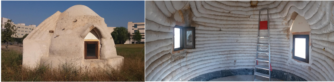
Fig. 1: Earthbag building, University of Lleida Campus, Spain.
