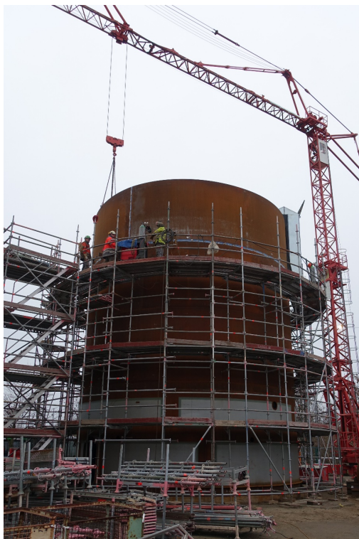
Figure 4: Buffer tank storage under construction (left) and finished (right) (pictures: Solites, 08.01.2020 and 16.06.2020)
