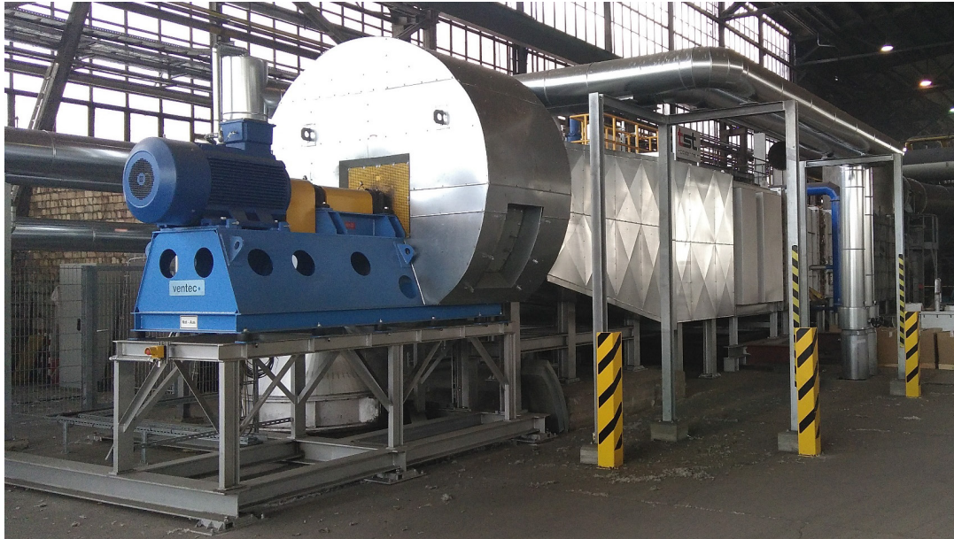
Figure 2: Heat exchanger subsystem to use industrial waste heat from steelworks (picture: Solites, 17.06.2020)
