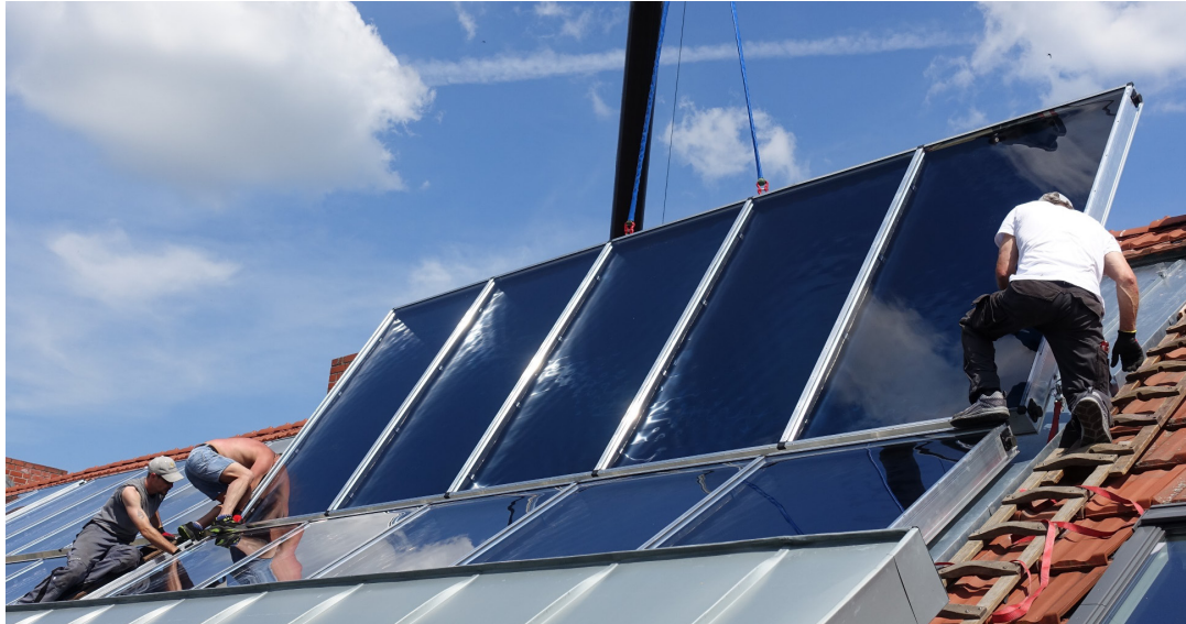
Figure 5: Replacement of formerly roof-integrated collectors on the roof of one out of five multifamily houses with large-scale solar thermal collectors on newly built sheet metal roof (picture: Solites, 17.06.2020)
